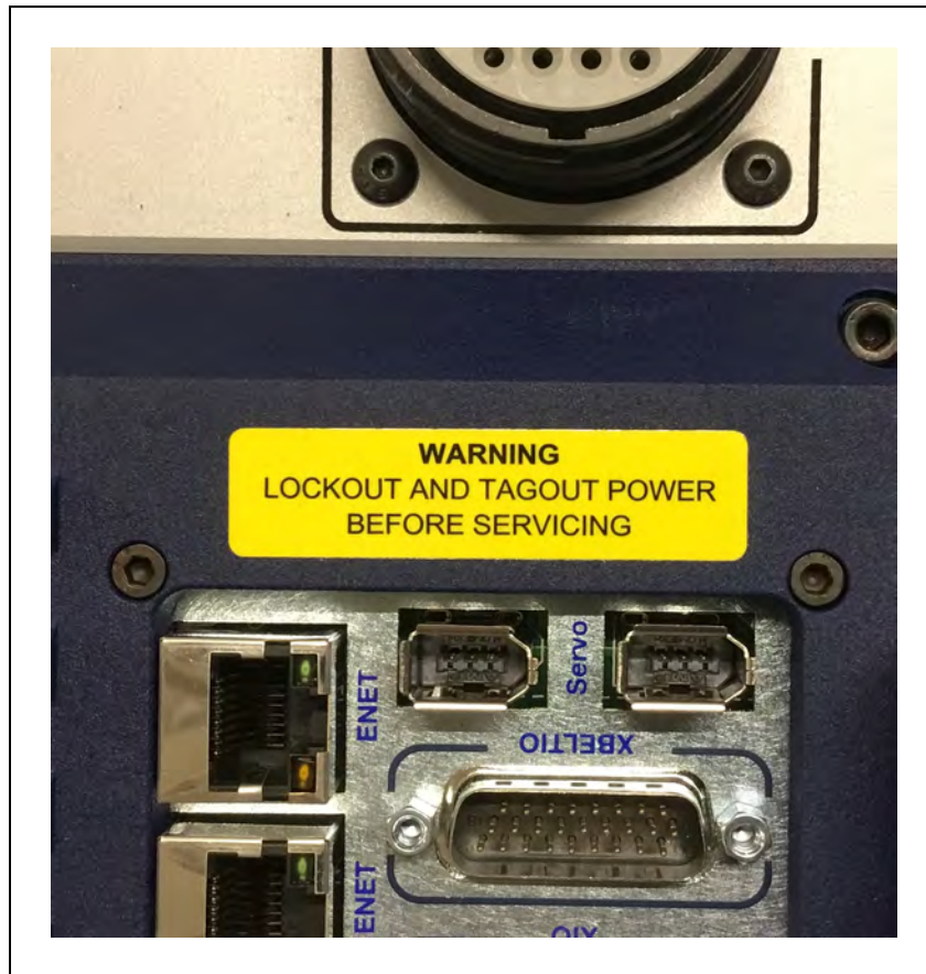
Figure 12-4. Lockout Tagout Warning Label
